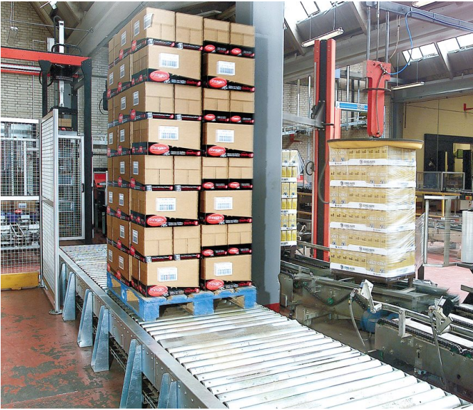
Pallet conveyor system at Dansk Kaffe Kompagni in Denmark.
